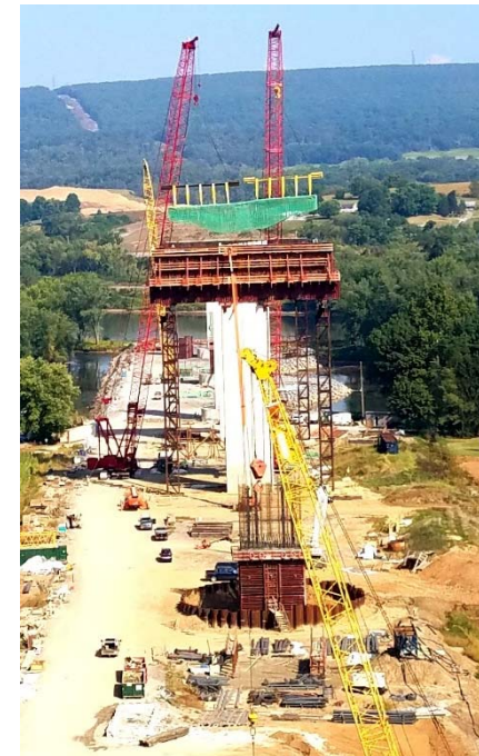
CSV T River Bridge (looking north across river)
