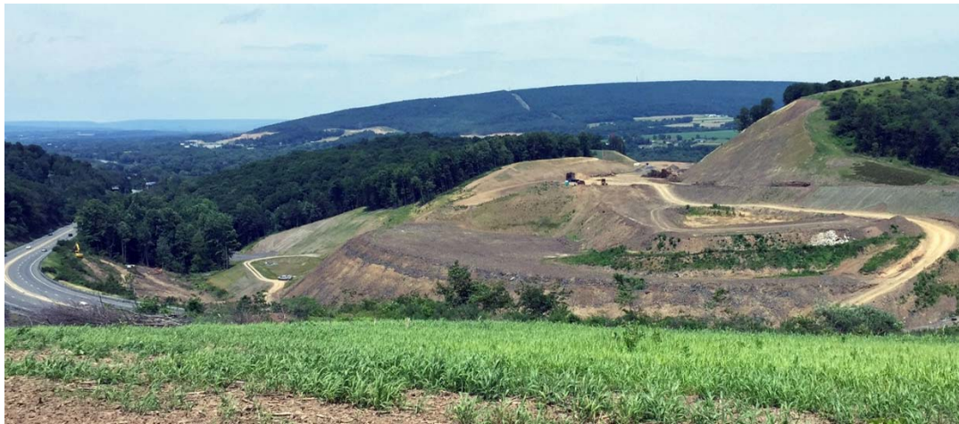
CSV T Northern Section (looking north across US 15 and river)
